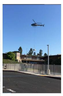
Units were craned onto the rooftop with a Helicopter because of challenges with site topography.
